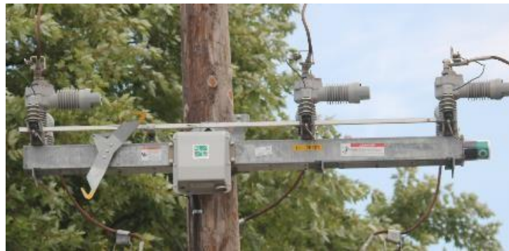
14 Figure 7: SCADA-Mate Switch
