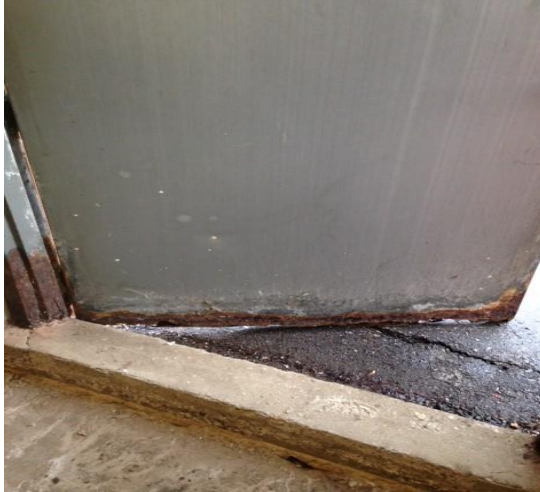
Figure 2: Rusted Door
