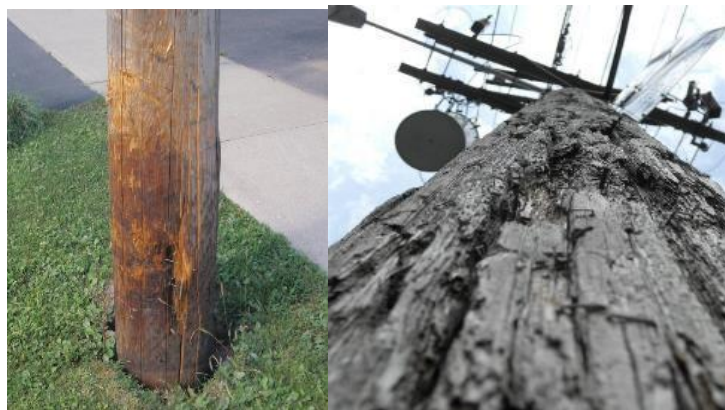
Figure 4: (Left) Cracked Wood Pole, (Right) Surface Rot on Pole
