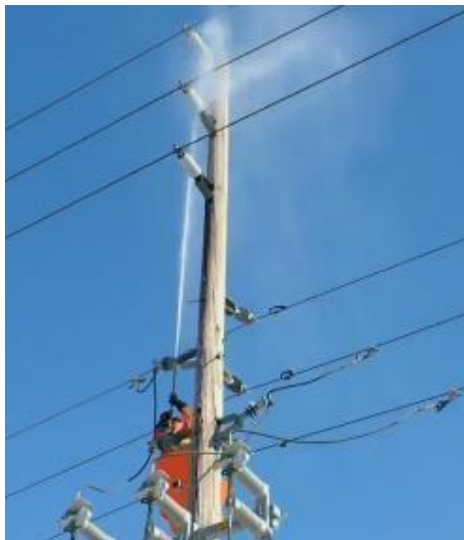
12 Figure 9: Porcelain Insulator Washed Using a High Pressure Water Jet
