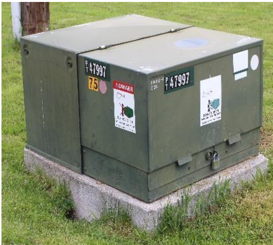
Figure 11: Padmounted Transformer
