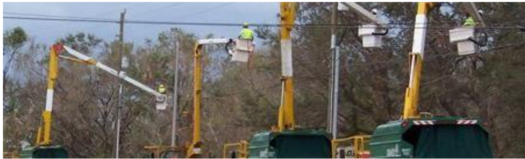
12 Figure 14: Tree Trimming of an Overhead Feeder
