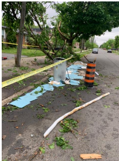
10 Figure 7: shows an Overhead Transformer taken down by a falling tree, spilling oil 11 onto the roadway and sidewalk (2022)
