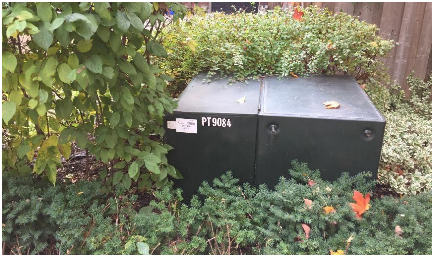
Figure 16: Padmounted Transformer Requiring Vegetation Removal
