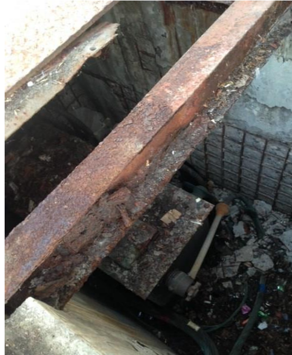
Figure 4: Corroded I-Beams
