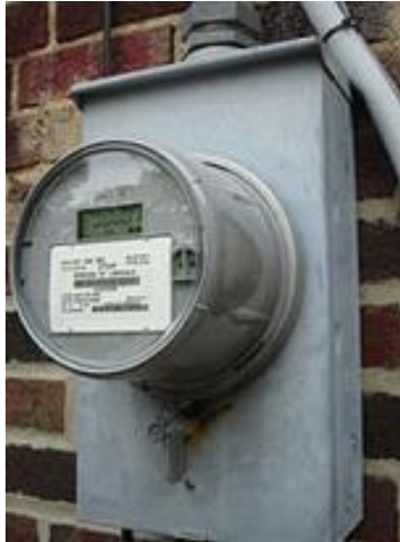
Figure 17: Smart Meter Installation at Customer Location.
