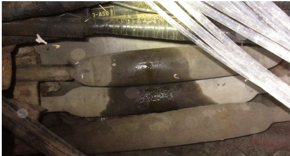
Figure 18: Oil Leakage from Cable Lead Splice
