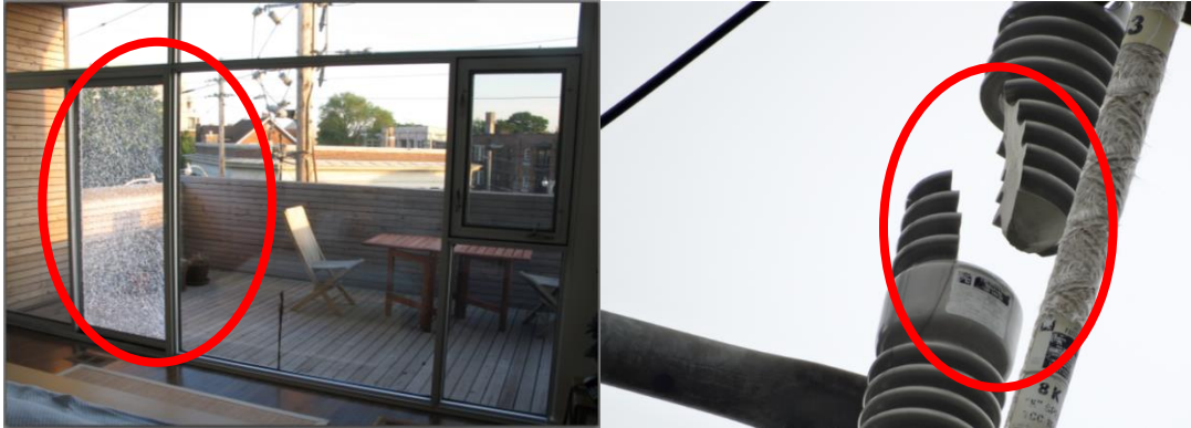
1 Figure 16: Porcelain Pothead Failure
