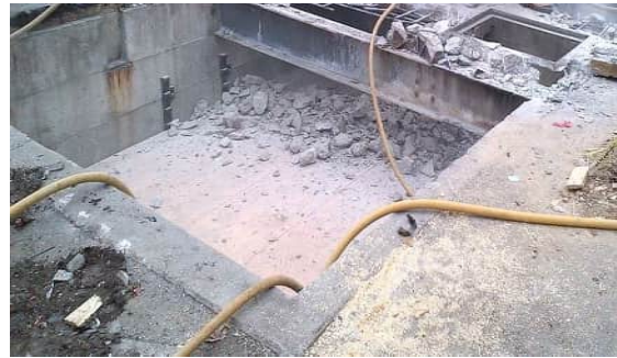
Figure 12: Temporary Roof during a Roof Rebuild
