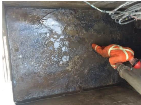
Figure 10: Deteriorated Vault Floor
