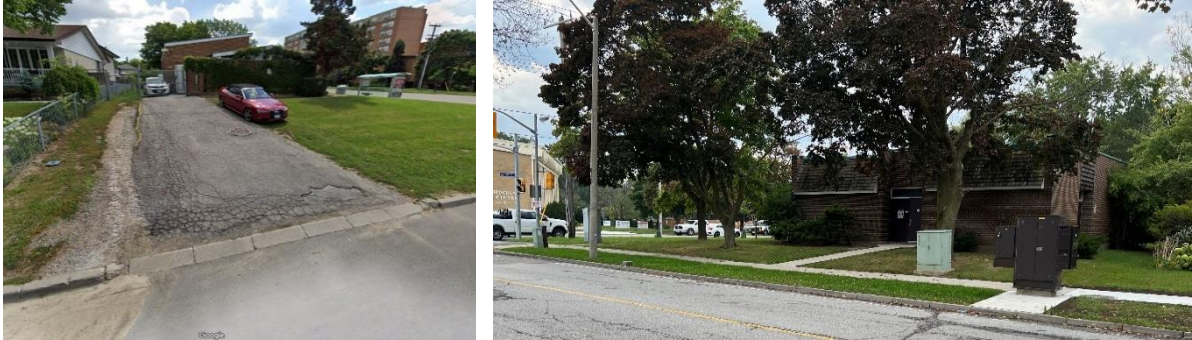
1 Figure 15: Examples of driveway deficiencies at Stations: Hunting Ridge Station driveway in 2 disrepair, Longfield Station with no available parking for response crews.
