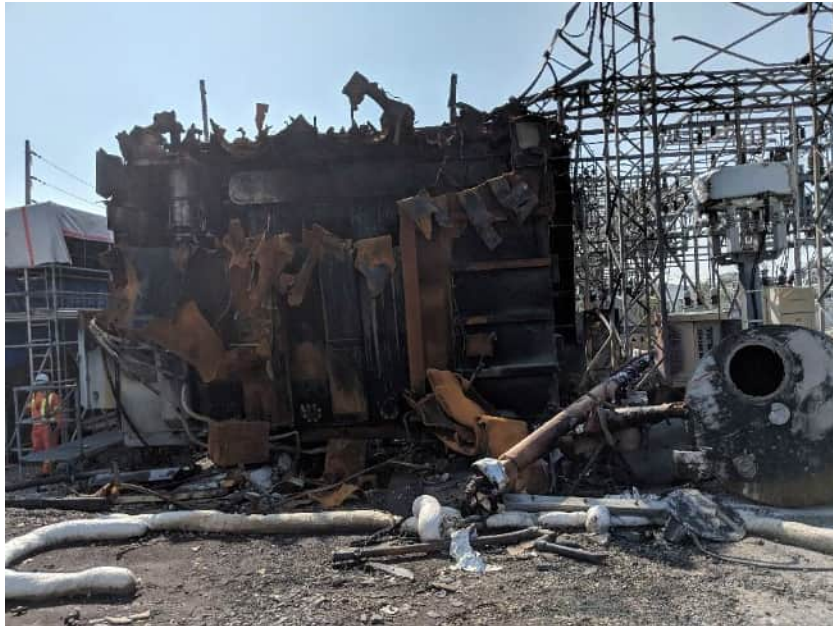
2 Figure 5: Post-Fire Damage at Finch Transformer Station Months Following a Major Event Day
