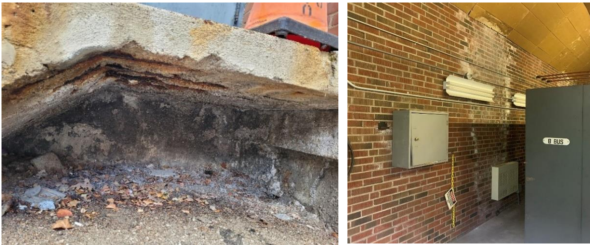
12 Figure 8: Examples of architectural deterioration at stations, from left to right: George and Duke 13 Station deteriorated concrete stairs, Centre Drive Station water infiltration from roof.
