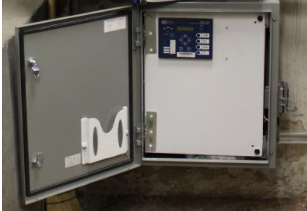
1 Figure 4: Toronto Hydro Communication Standard for DER Connections (left) and Communication 2 Gateway Installed at Customer DER Site
