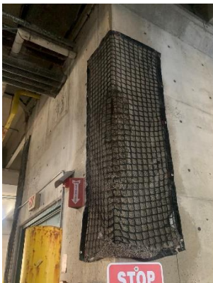
7 Figure 5: Examples of structural deterioration at work centres, from left to right: 500 8 Commissioners Building C – spalling concrete wall with preventative netting; 500 Commissioners 9 Building C – exposed deteriorated waterproofing; 500 Commissioners Building C – rusted steel 10 staircase.
