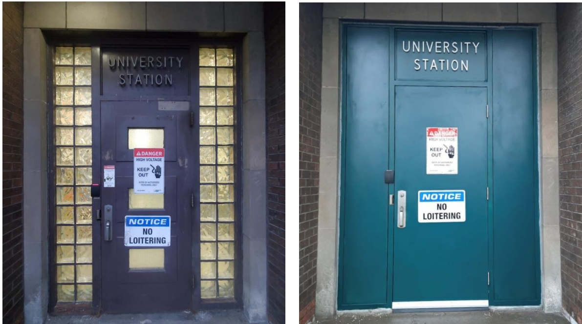
1 Figure 18: Examples of University Station entrance door in poor condition (left) and after being 2 retrofitted via the station door program (right).
