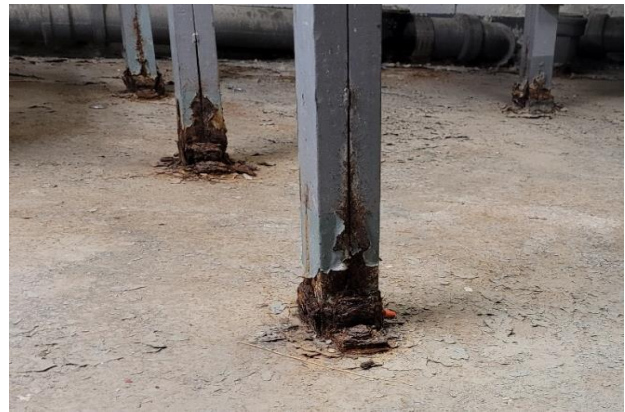
2 Figure 4: Examples of structural deterioration at stations, from left to right: Windsor Station 3 cracked concrete floor slab, Windsor Station corroded rebar columns.
