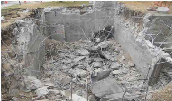
Figure 11: In-Progress Vault Decommissioning
