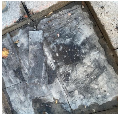
7 Figure 5: Examples of structural deterioration at work centres, from left to right: 500 8 Commissioners Building C – spalling concrete wall with preventative netting; 500 Commissioners 9 Building C – exposed deteriorated waterproofing; 500 Commissioners Building C – rusted steel 10 staircase.
