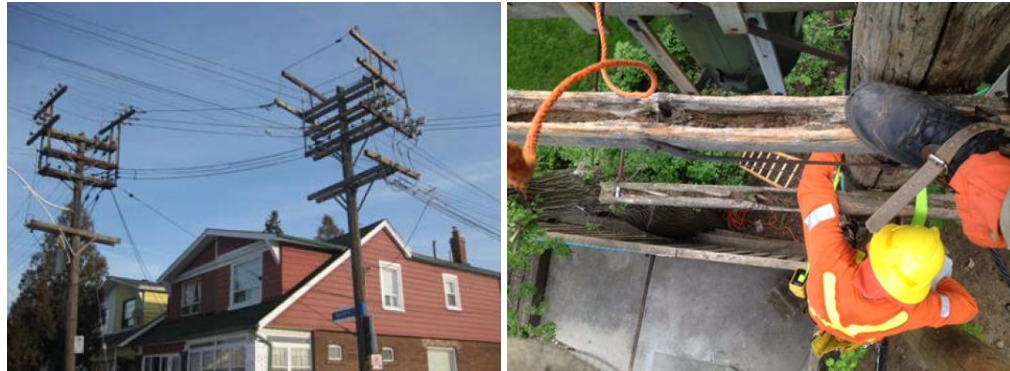
1 Figure 8: Box Construction (left). Replacing a transformer on a 2 poor condition Rear Lot pole (right)
