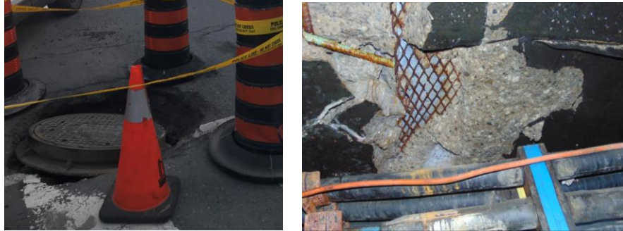
1 Figure 14: Cable Chamber Roof in HI5 Condition (Left), and Roof Inside View (Right)
