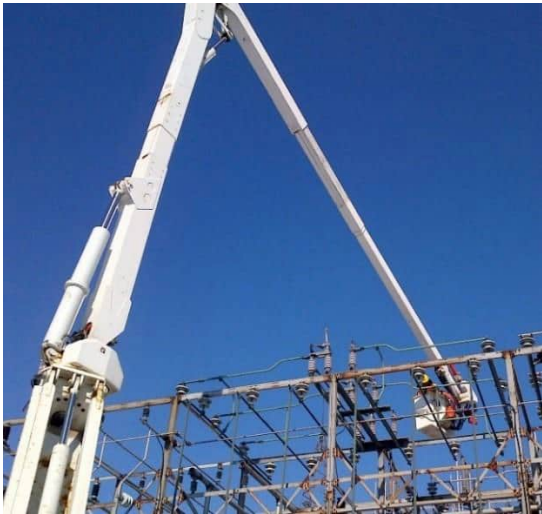
Figure 13: Repair of TS Outdoor Switch
