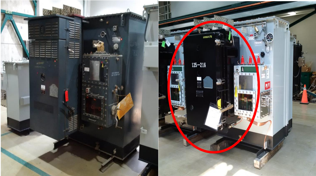
1 Figure 26: A ventilated Network Unit (Left) and a Submersible Network Unit (Right)
