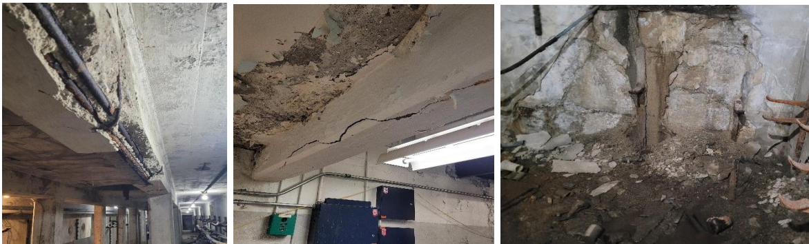
14 Figure 16: Examples of existing stations in critical condition, from left to right: George and Duke 15 Station, beam with exposed rebar, Defoe Station cracked beam, Junction Station deteriorated 16 foundation wall.
