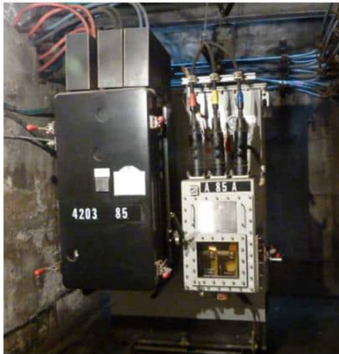
Figure 7: An Example 500 kVA Network Unit
