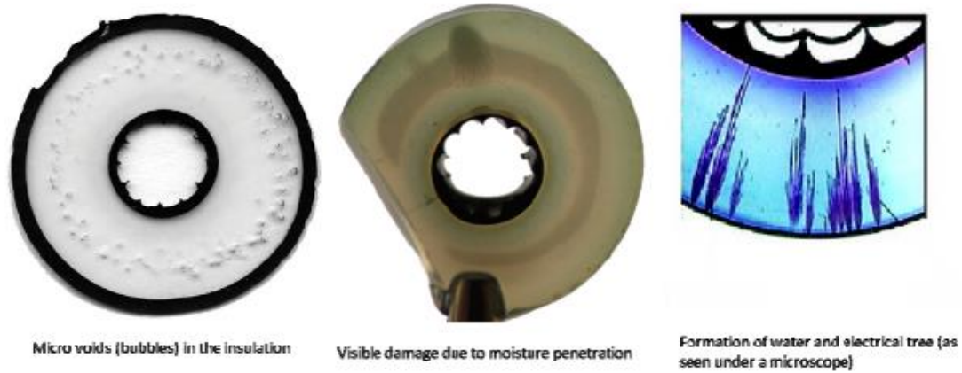
Figure 22: Field and Laboratory Sample of Microscopic Voids and Damage XLPE Insulation
