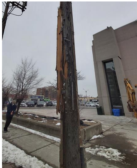
9 Figure 1: Pole struck by vehicle identified through a patrol
