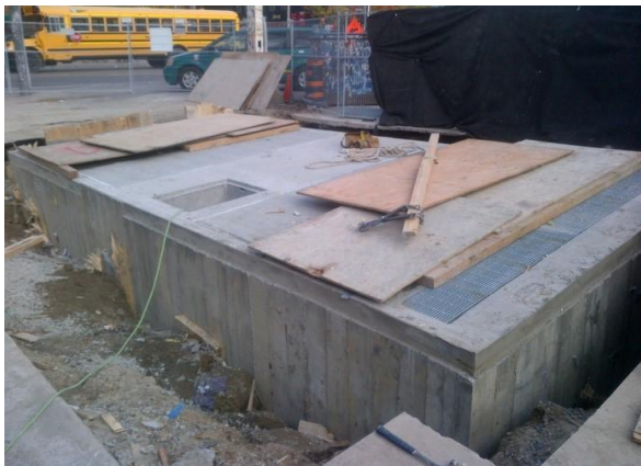
Figure 13: Completely Rebuilt Vault
