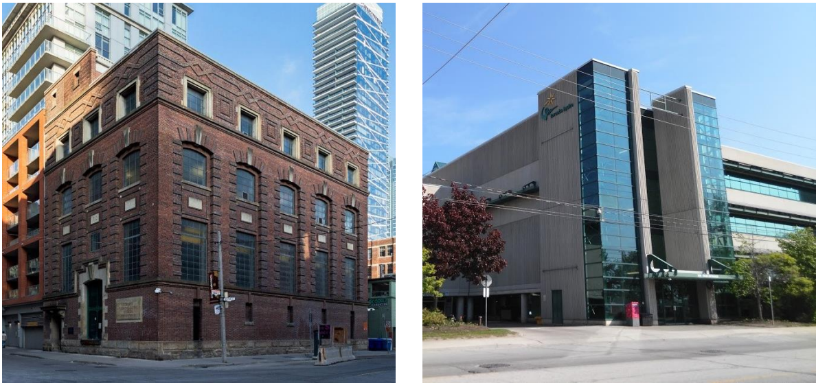
9 Figure 1: Examples of Toronto Hydro infrastructure; a downtown substation and work centre.
