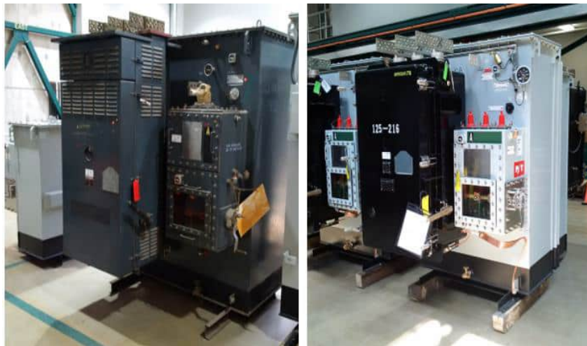
14 Figure 1: Snapshot of a Ventilated Network Unit (L) and Submersible Network Unit (R). The black 15 protector is of a submersible design, which prevents water ingress.
