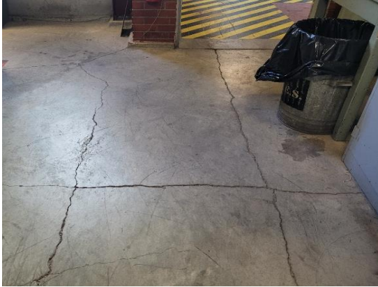
2 Figure 4: Examples of structural deterioration at stations, from left to right: Windsor Station 3 cracked concrete floor slab, Windsor Station corroded rebar columns.
