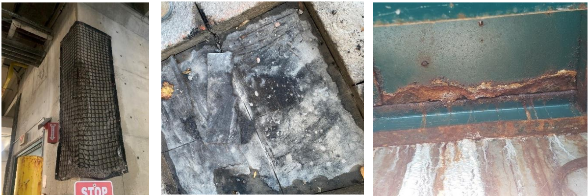
7 Figure 5: Examples of structural deterioration at work centres, from left to right: 500 8 Commissioners Building C – spalling concrete wall with preventative netting; 500 Commissioners 9 Building C – exposed deteriorated waterproofing; 500 Commissioners Building C – rusted steel 10 staircase.
