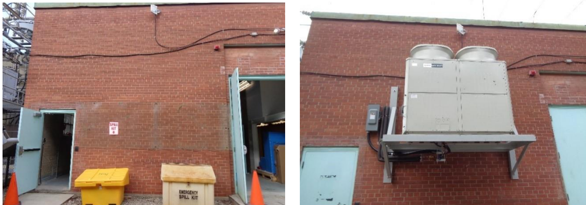
9 Figure 13: Examples of HVAC additions at Stations: Strachan Station without additional air 10 conditioning (left) and after with two new condensing units installed for keeping air temperature 11 and equipment cool (right).
