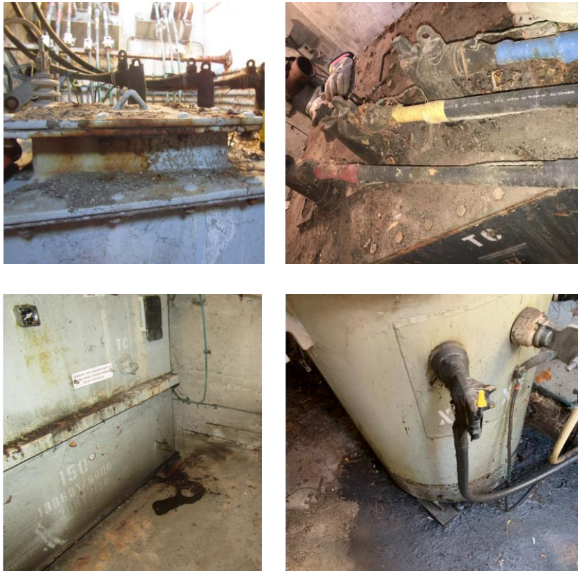
1 Figure 32: Examples of URD Transformers Exhibiting Corrosion on Lids and Oil Leaks
