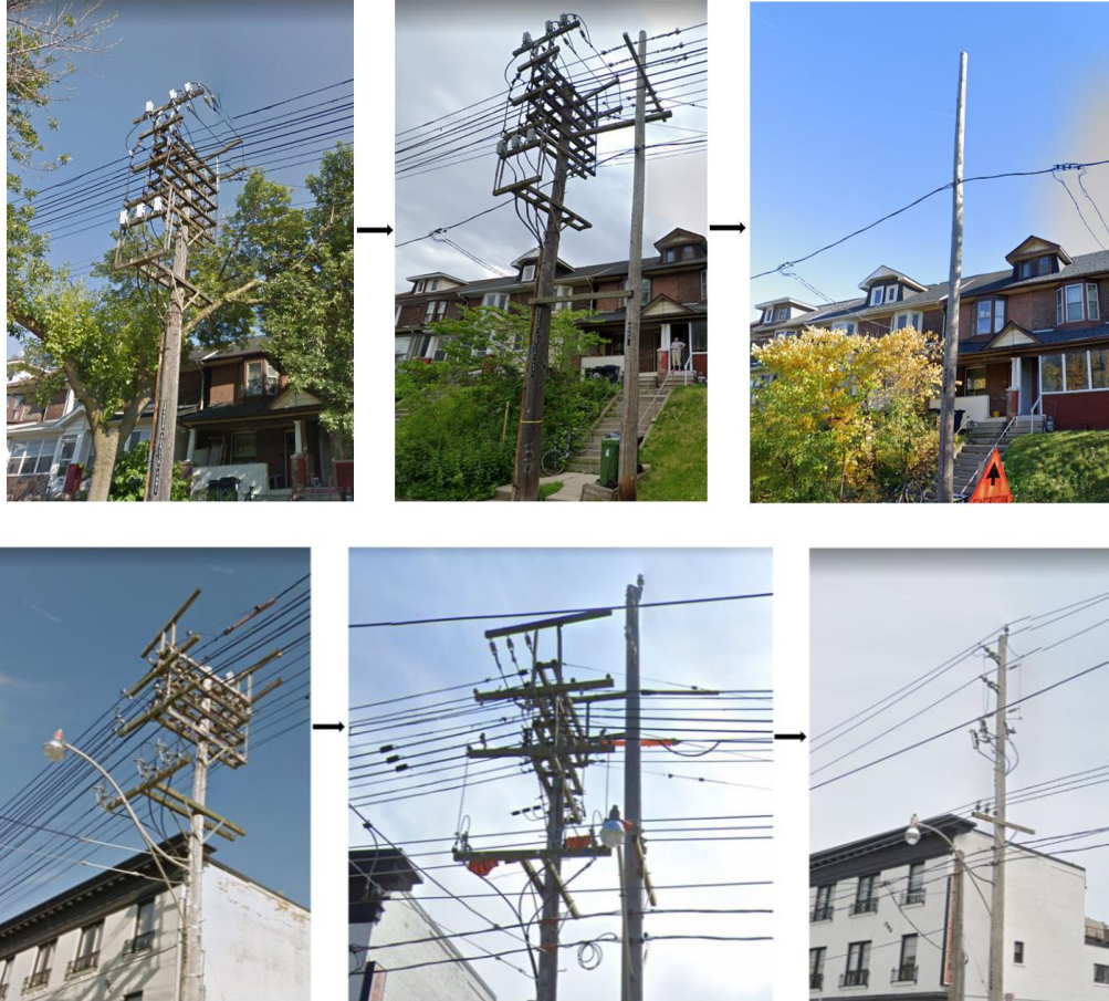
1 Figure 10: Actual box construction conversion project on Gerrard Street East at two locations. 2 Photographs on the left show 4.16 kV box construction poles prior to conversion. Photographs in 3 the middle are demonstrating the in-construction stage. The completed project is shown in the 4 photographs on the right, where all 4.16 kV box construction has been removed.
