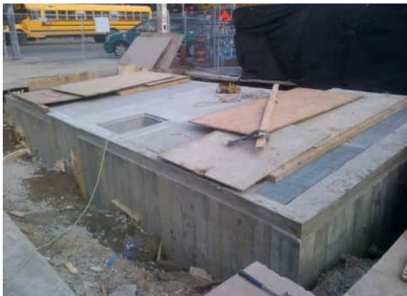
Figure 13: Completely Rebuilt Vault
