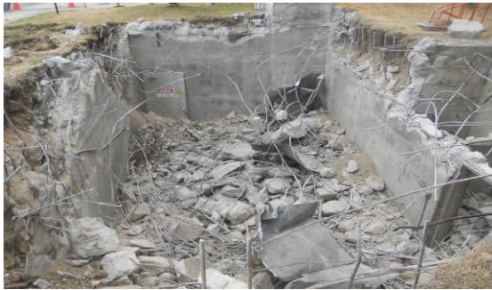
Figure 11: In-Progress Vault Decommissioning
