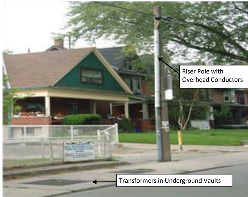
1 Figure 18: Typical Layout of Underground Residential Distribution
