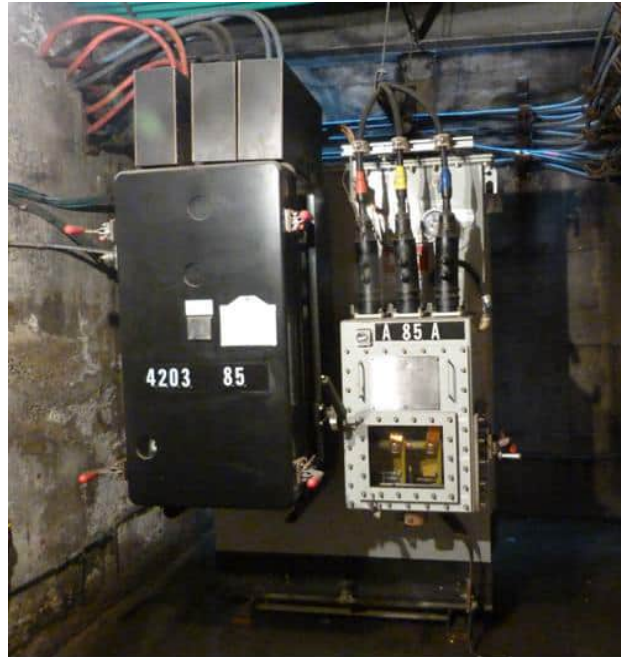
Figure 23: Submersible Network Unit
