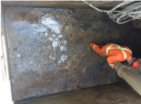
Figure 10: Deteriorated Vault Floor
