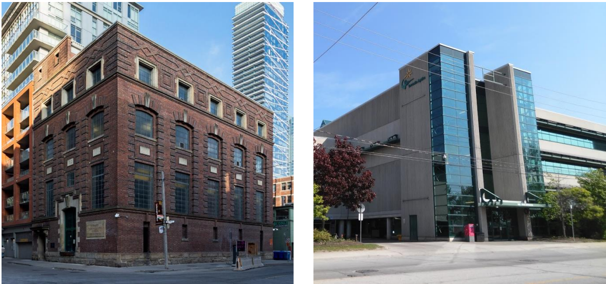
9 Figure 1: Examples of Toronto Hydro infrastructure; a downtown substation and work centre.
