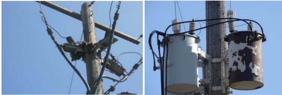
6 Figure 10: Animal Contact on Metal Switch Bracket (Left)/Rusted Overhead Transformers at Risk of 7 Leaking Oil (Right)
