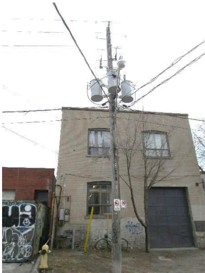
P27 OT24584 – 3-PH Transformer Installation
