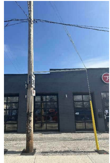
P50 – Pole Installation (Stenciling Issue Fixed)
