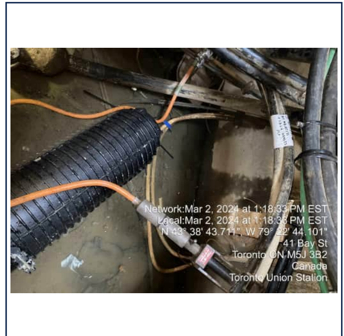
Spike Tool Installed
