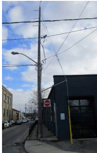
P11 (Existing Pole) – Guying Installation
