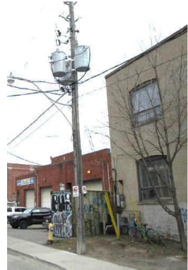
P27 – Guying Installation
