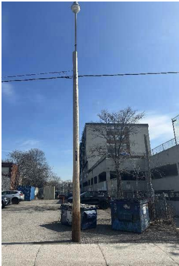
P20 – Pole Installation (Secondary Conductor and Stenciling Issues Fixed)
