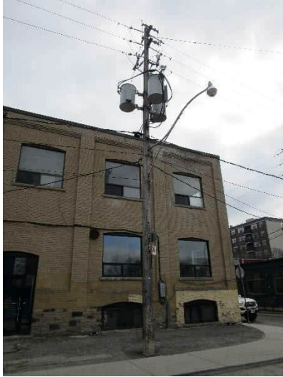
P58 OT400445 (Existing) – 3-PH Double Dead-End Configuration
