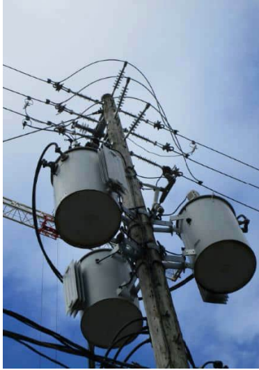
P58 OT400445 – Overhead Conductors Installation
