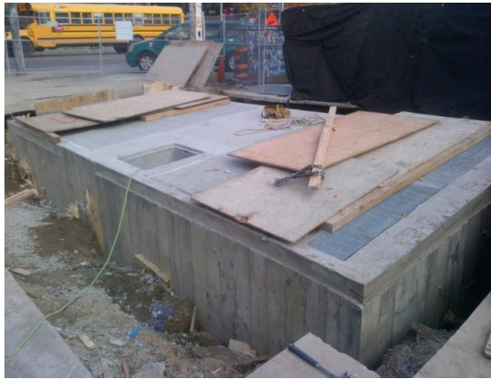
Figure 10: Completely Rebuilt Vault
