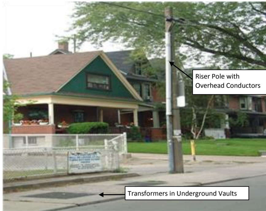
1 Figure 13: Typical Layout of Underground Residential Distribution
