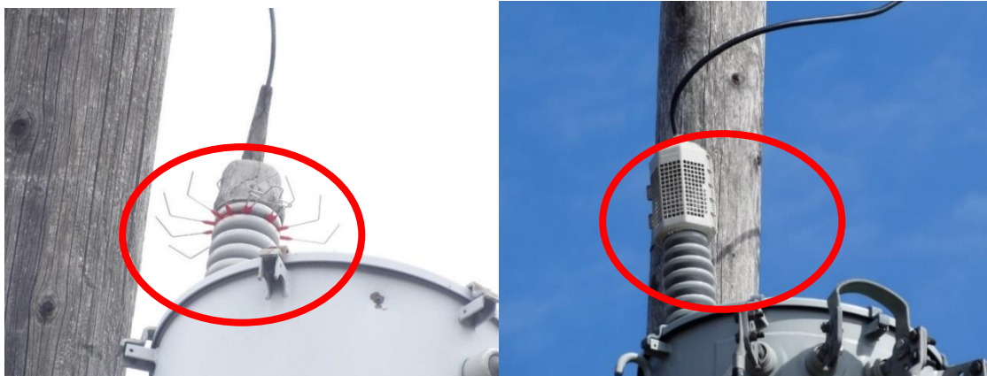
Figure 12: Animal Guards – Guthrie Guard (left), Newer Wildlife Guard (Right)
