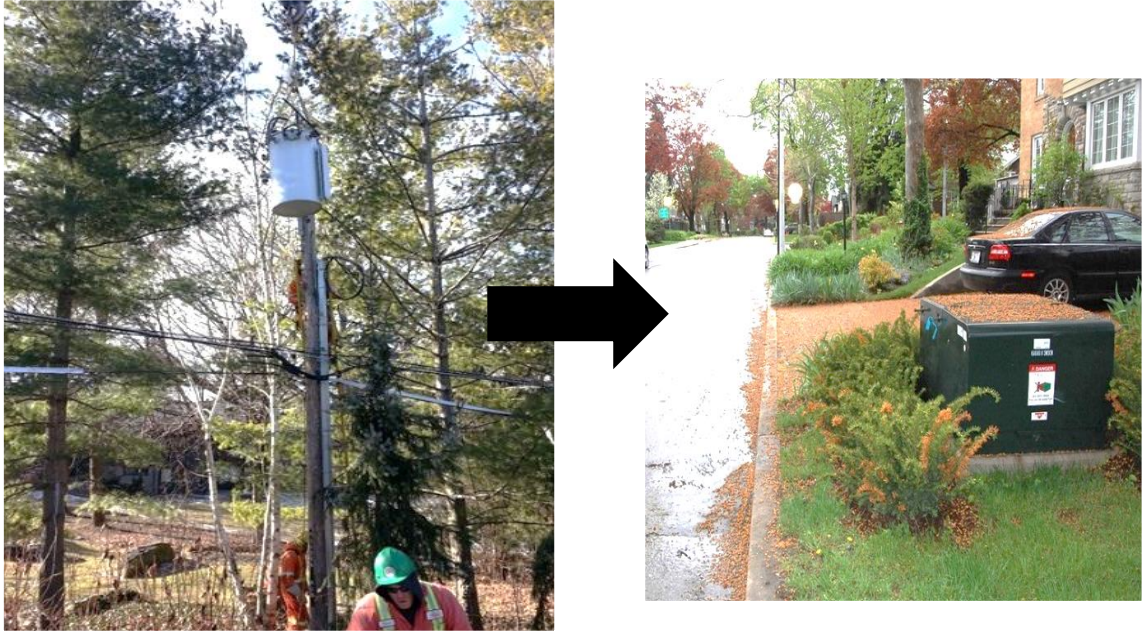
1 Figure 1: Legacy rear lot supply vs. replacement front lot supply.
