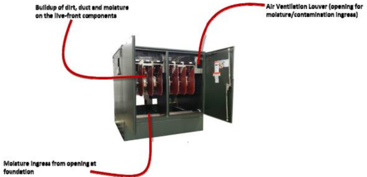
Figure 16: Padmounted switch
