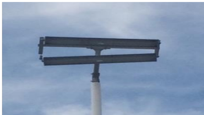
10 Figure 7: Blown yard light hanging by an electrical wire
