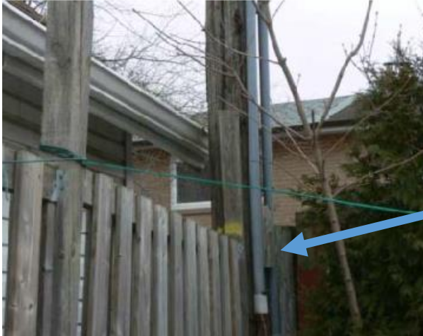
1 Figure 8: Fence built on easement and exposed cable from broken guard
