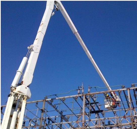
Figure 13: Repair of TS Outdoor Switch
