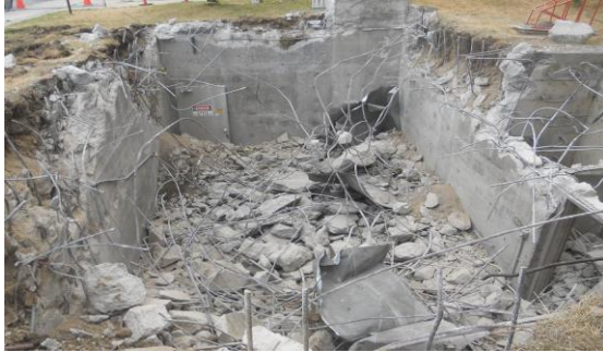
Figure 8: In-Progress Vault Decommissioning
