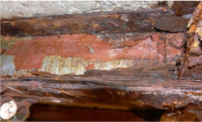
Figure 14: Corroded I-beams
