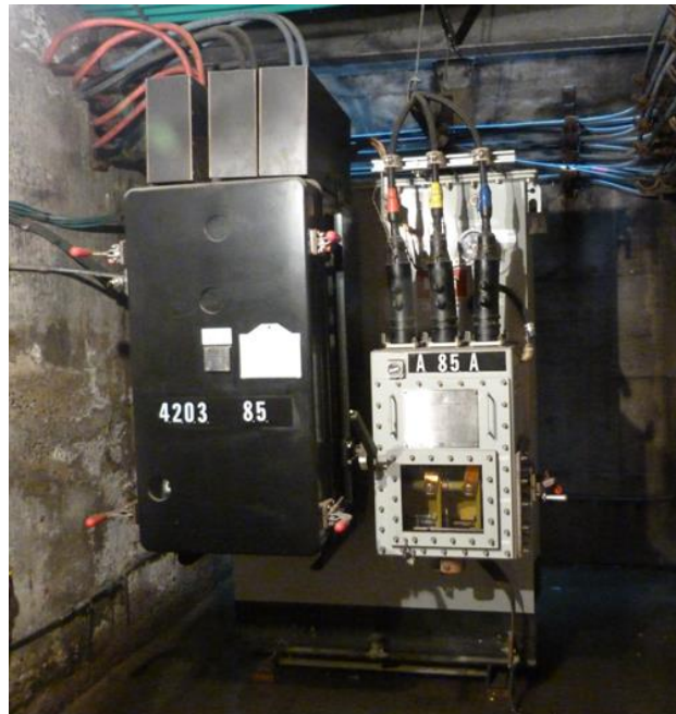
Figure 18: Submersible Network Unit
