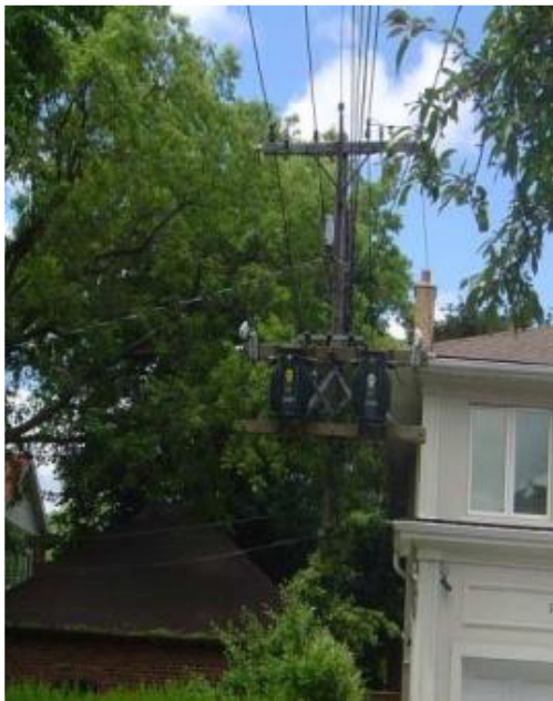
14 Figure 7: Energized transformer and pole line close to home and covered in vegetation
