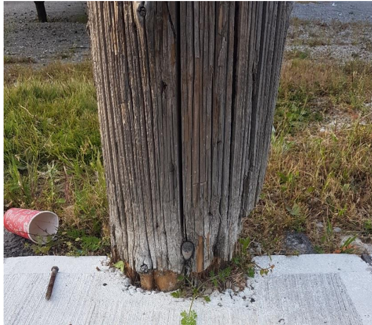
Figure 12: Deterioration at the base of a pole
