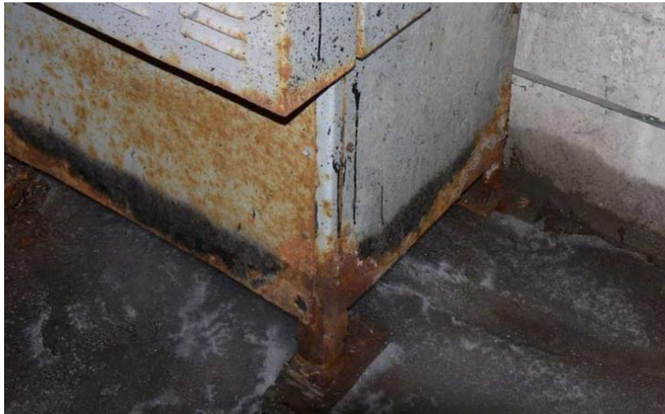
Figure 1: Rusting at Base and Footing of ATS Unit
