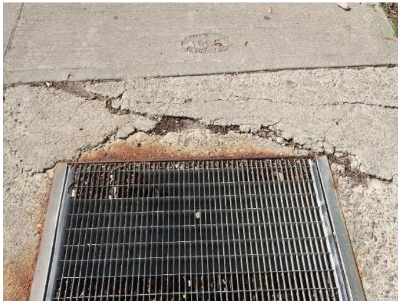
Figure 22: URD Vault with Deficient Roof
