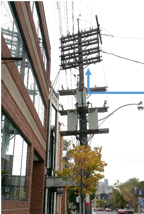
Figure 10: Example of Box Construction clearance issues
