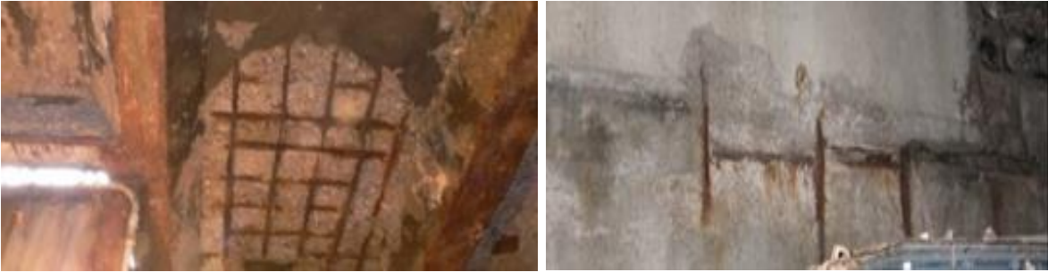
Figure 13: Roof and wall with exposed rebar
