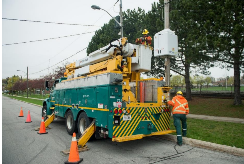
4 Figure 9: Installation of Pole-Mounted Energy Storage Systems
