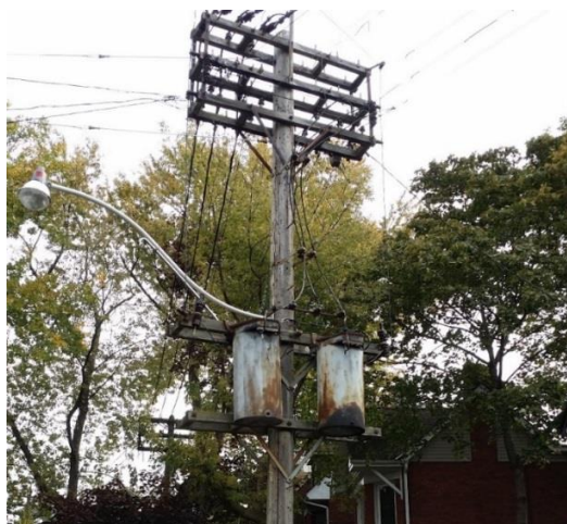
Figure 4: Box Construction in a Backyard with Leaking Equipment
